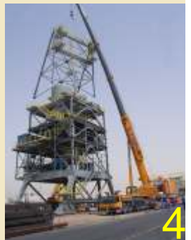
SOHAR ALUMINIUM PROJECT 800 t/h ship unloader 8
