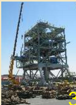
SOHAR ALUMINIUM PROJECT 800 t/h ship unloader 8
