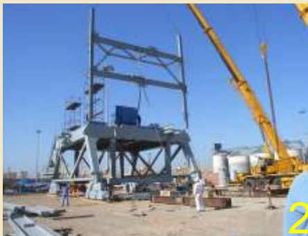
SOHAR ALUMINIUM PROJECT 800 t/h ship unloader 8
